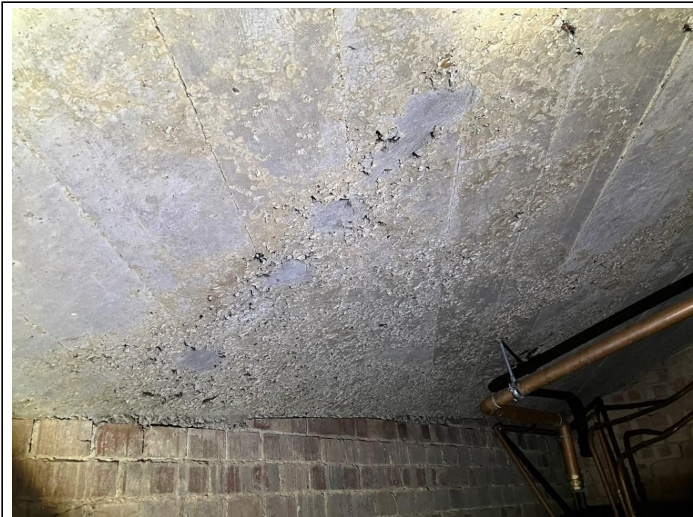
23. Loft space, spalling concrete.
