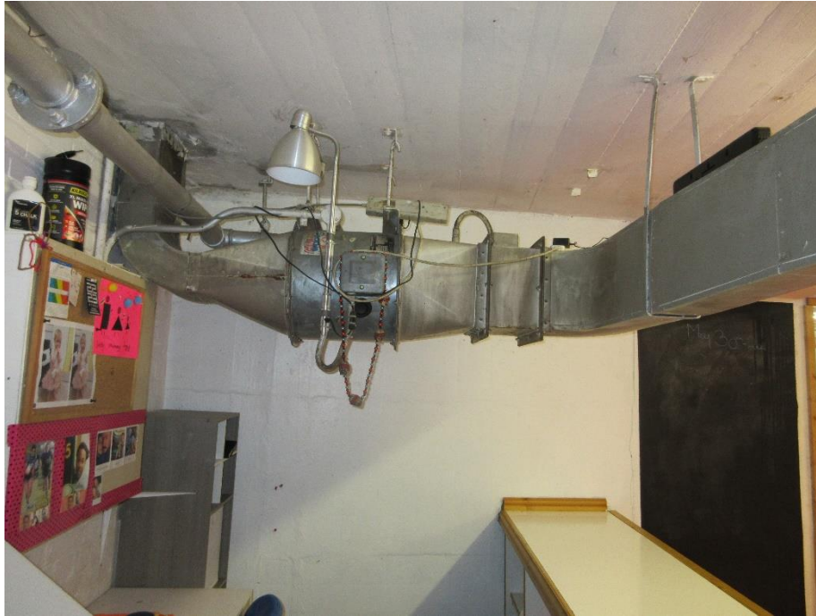
53. Extract fan serving the basement
