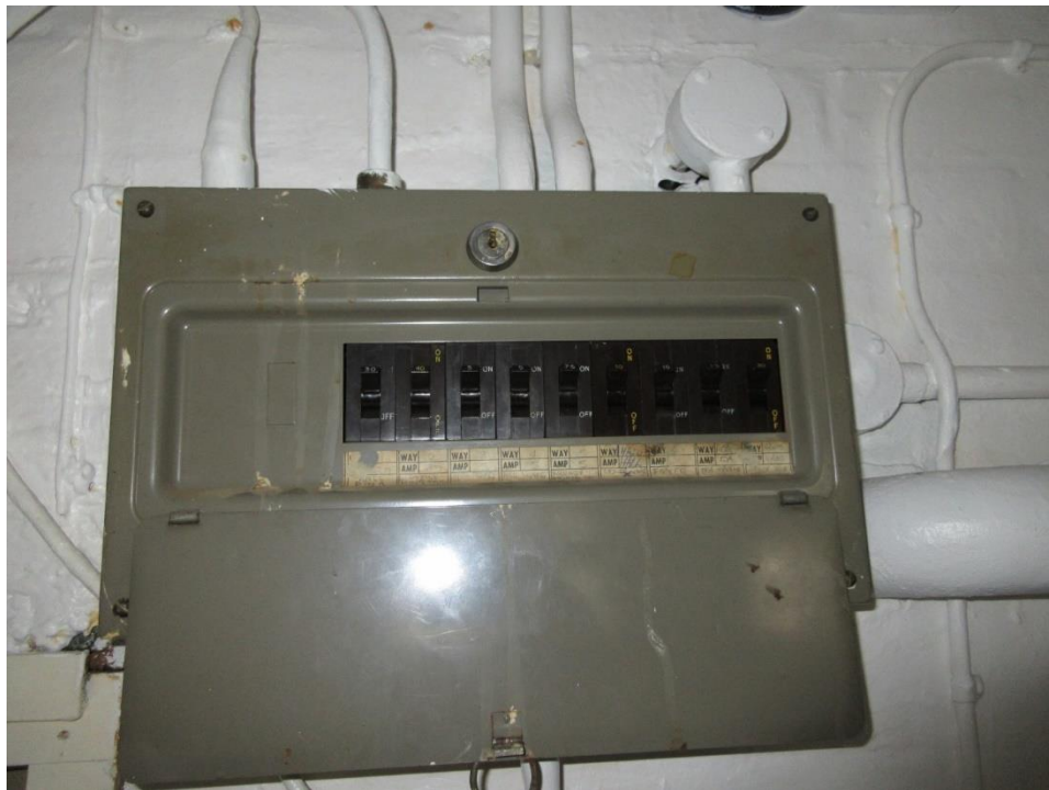
65. Typical aged distribution board, no circuit schedule
