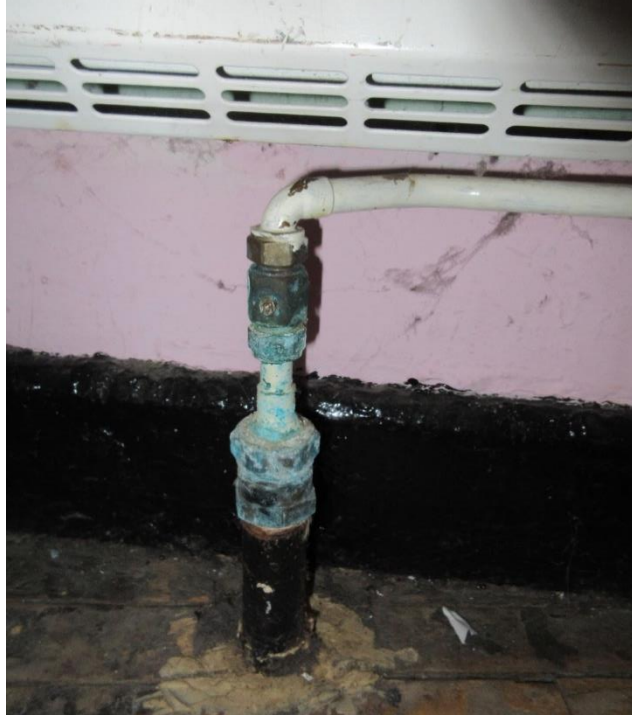
56. LTHW connections on the LST radiators are exposed and some are show signs of leaks / corrosion
