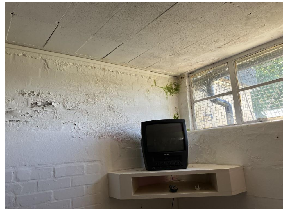
30. Ground floor east section, stained painted masonry wall.
