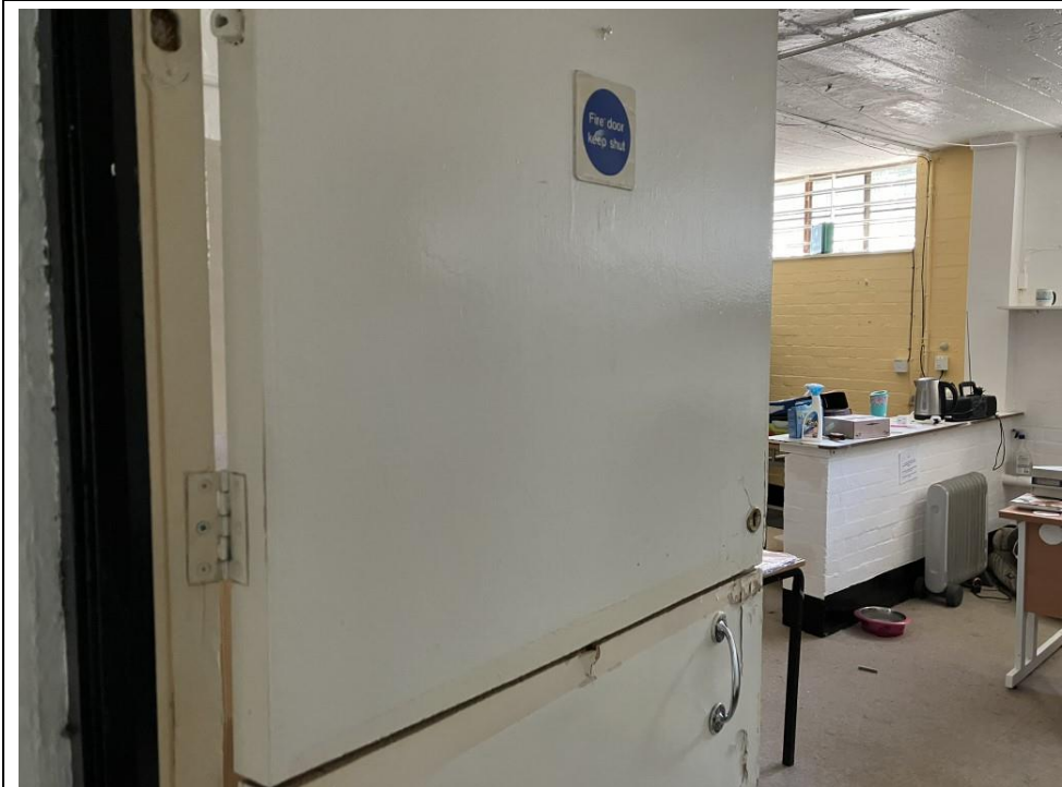
42. Ground floor east section, fire door compromised to form a "Dutch" Door.
