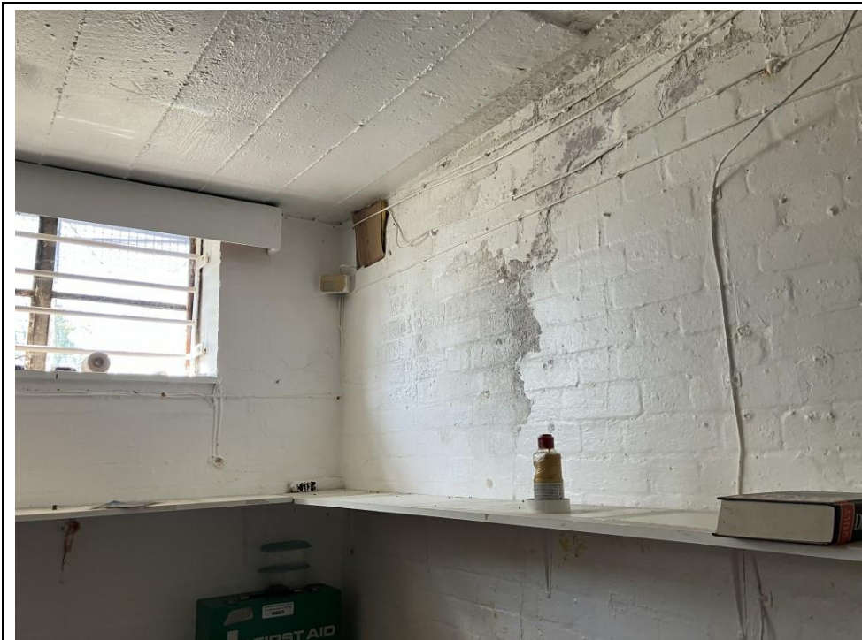
29. Ground floor east section, stained painted masonry wall.
