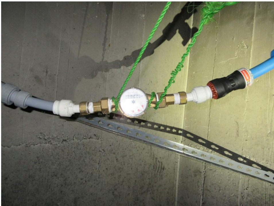
59. Poorly supported check meter on the mains water service at basement level, resulting in excessive pressure applied to connections
