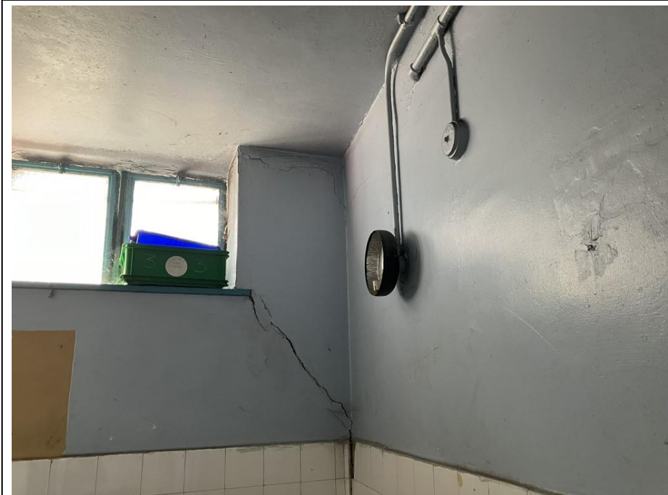
32. Ground floor central section, moderate crack.
