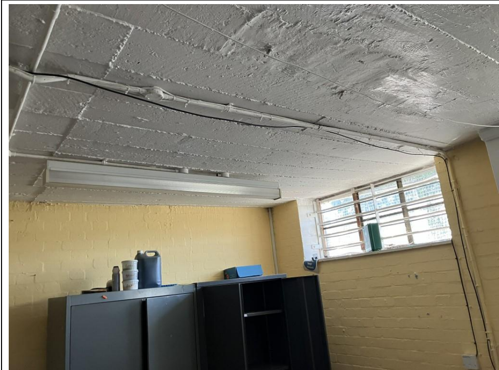
24. Ground floor east section, typical painted concrete board ceiling.
