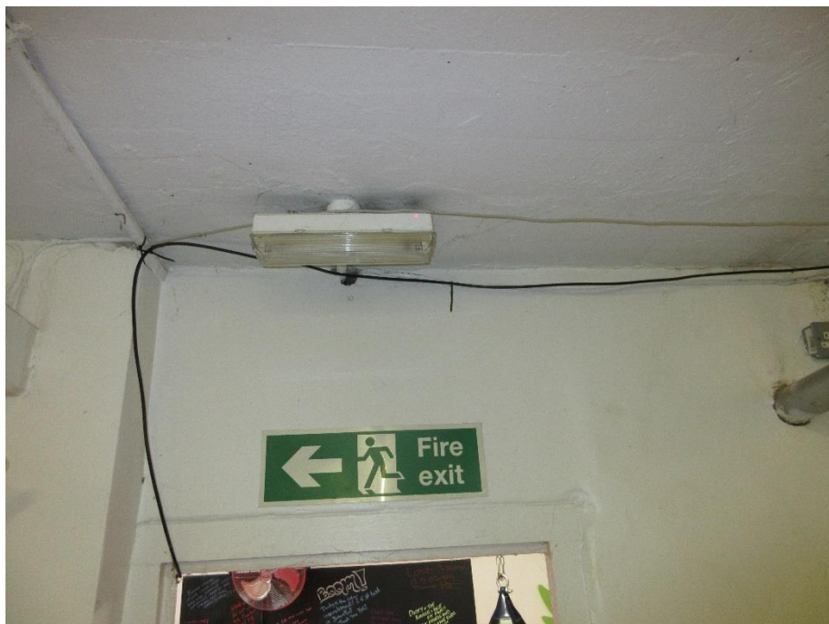
68. Typical emergency light, emergency lighting and signage should be reviewed on site and additional service provided where required
