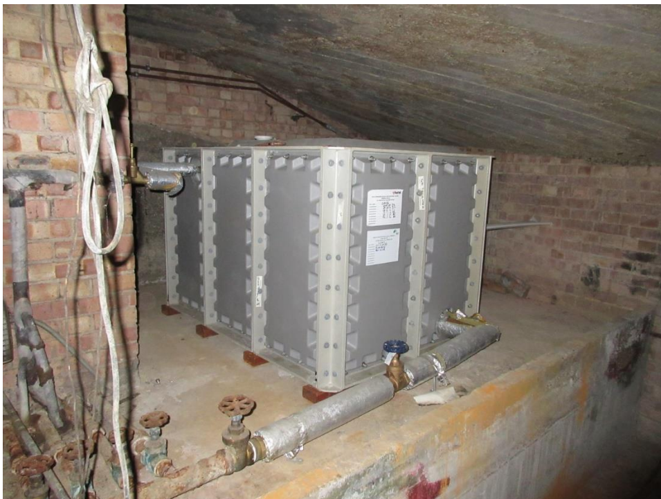
60. Cold water storage tank in the roof void
