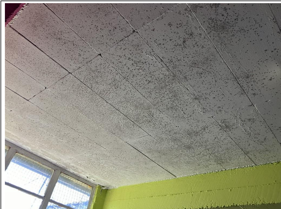
25. Ground floor east section, typical mould growth.
