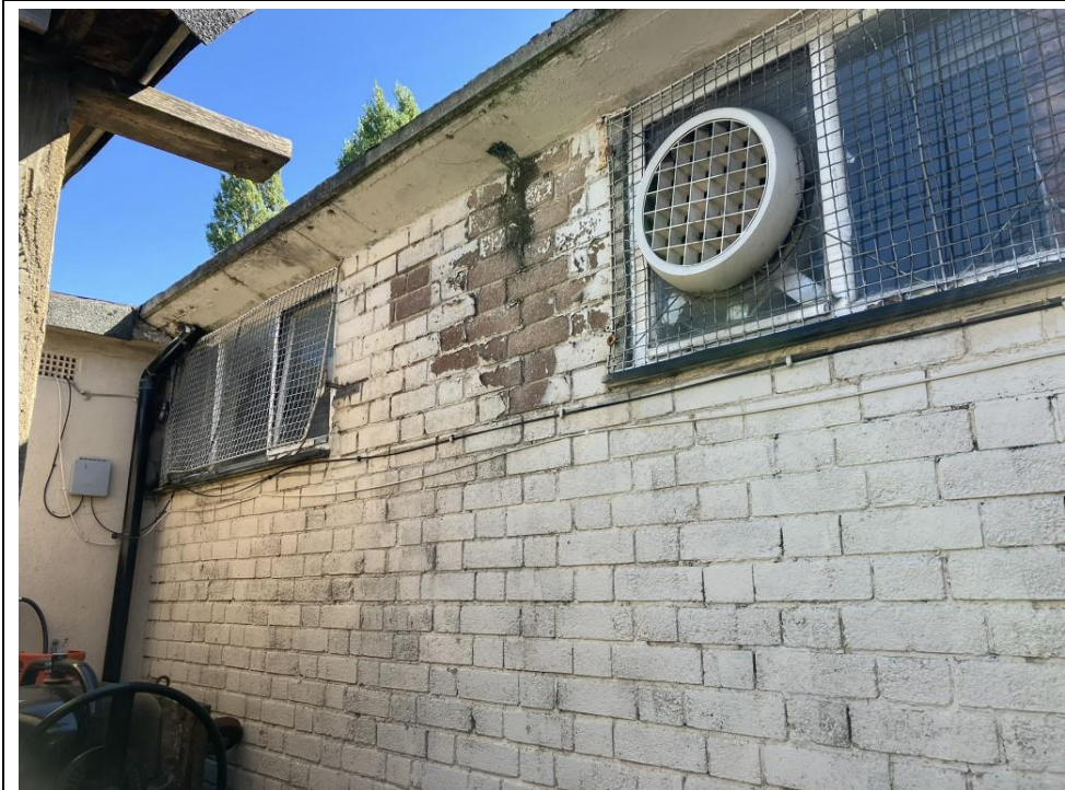
13. Rear elevation west section, missing rainwater outlet.
