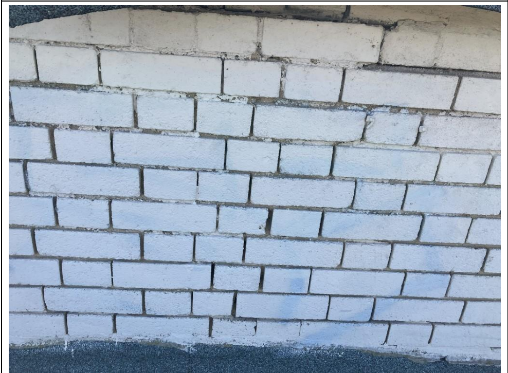
9. Central section (roof level), indicative failed pointing.
