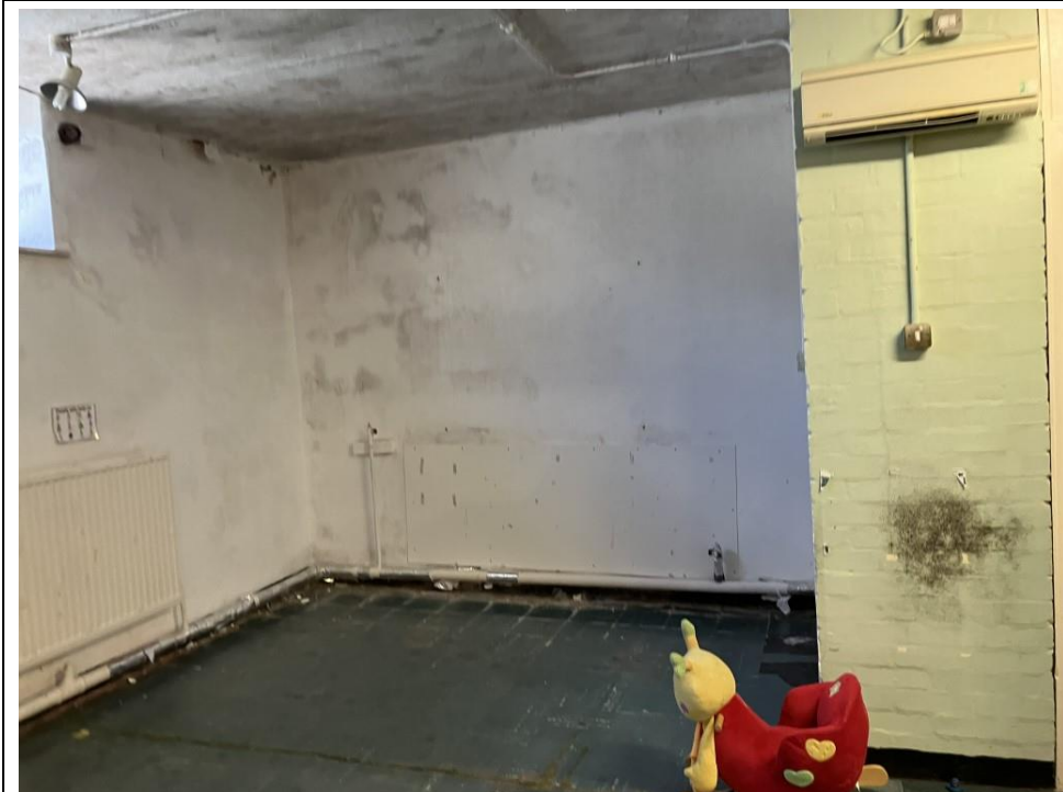
36. Ground floor west section, indicative mould growth and staining.
