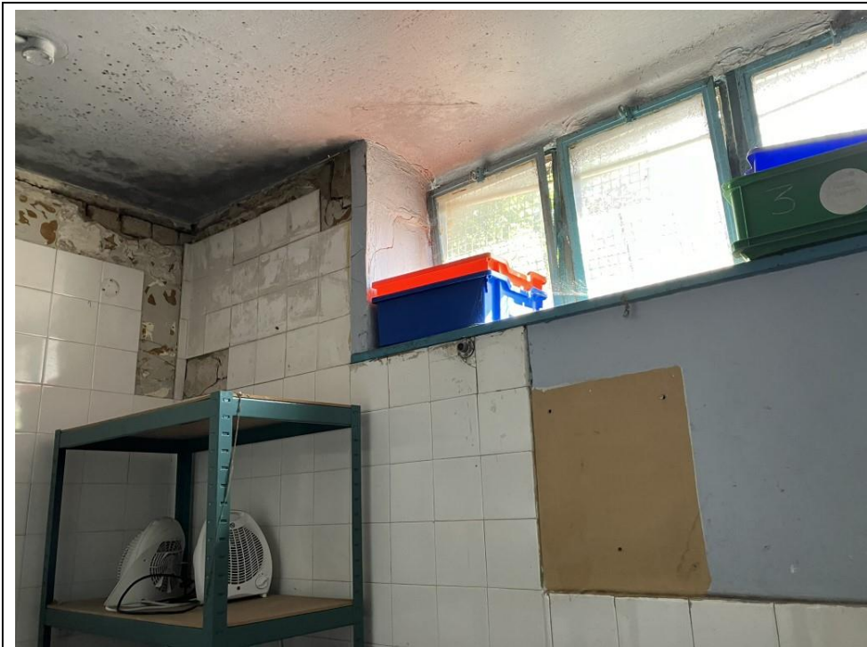
33. Ground floor central section, failed wall tiles.
