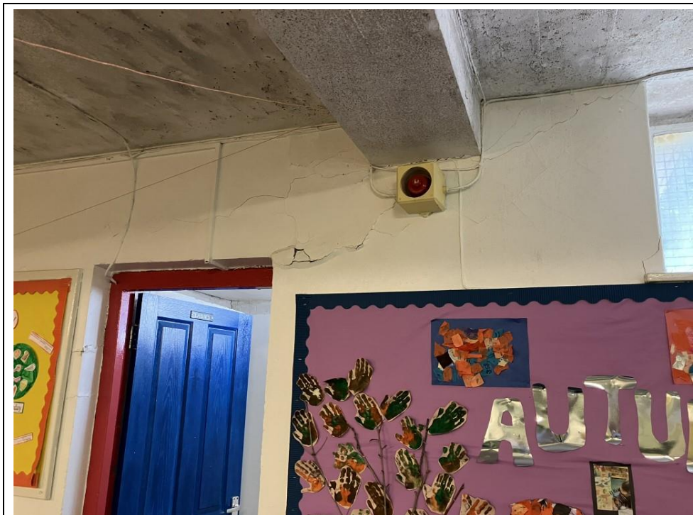
37. Ground floor west section, indicative cracking.
