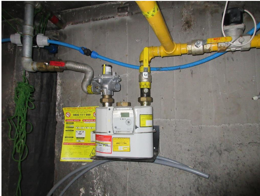
51. Incoming gas service, utility meter and solenoid valve within the basement plant room.
