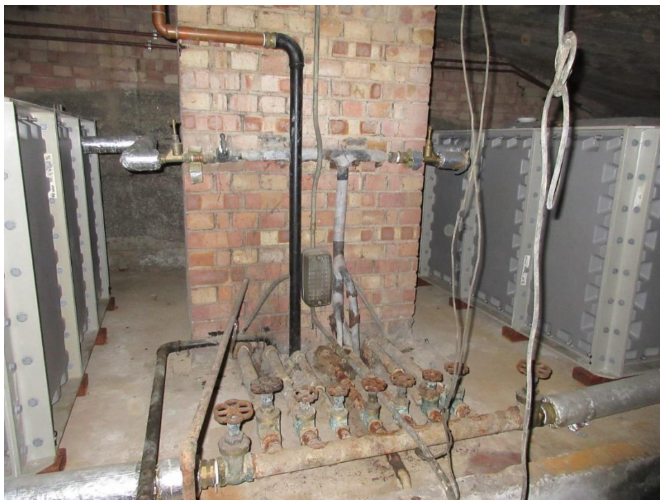
61. Mixture of pipework materials, lead, copper, steel
