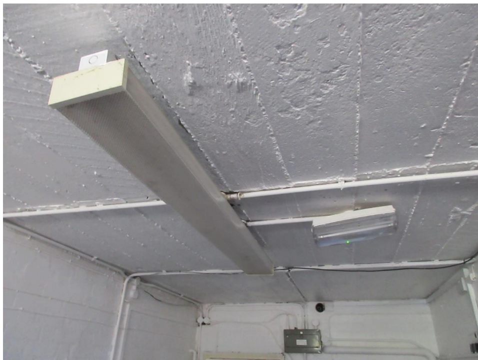
66. Typical aged fluorescent lighting and emergency lighting
