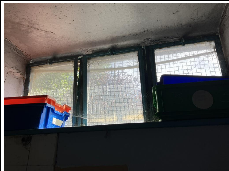
41. Ground floor central section, typical Crittall style window.
